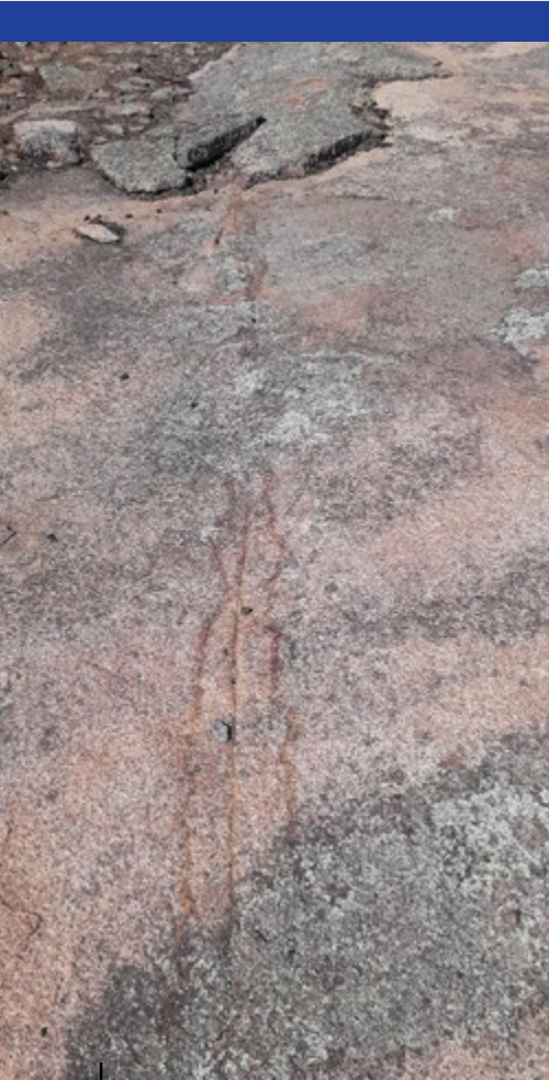
Fracture in granite pavement at Arthur River possibly related to seismic activity.
